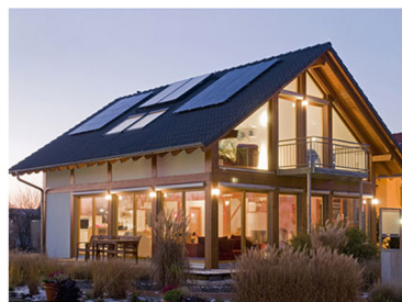
Off grid power system
