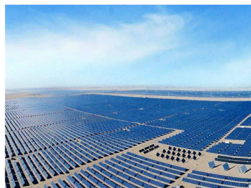
Photovoltaic power station
